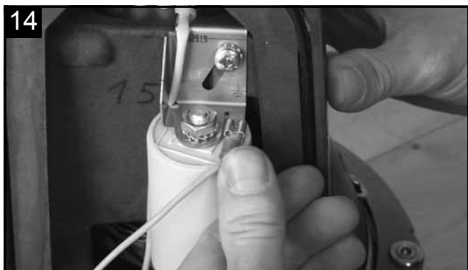
Fit the earth lead on the new bracket
